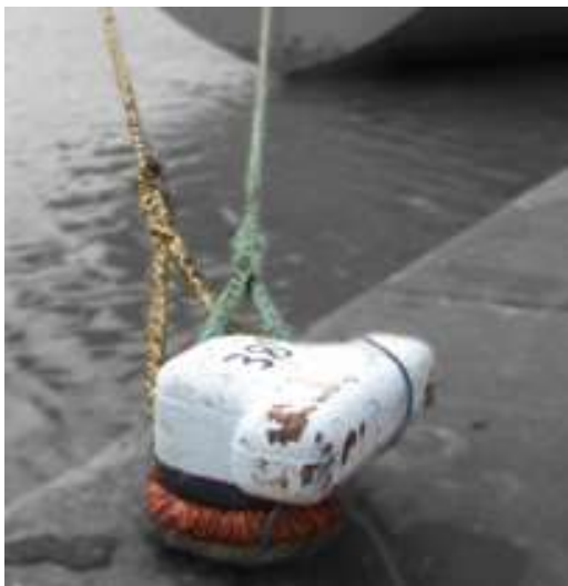
Fig 3: A conventional mooring bollard
