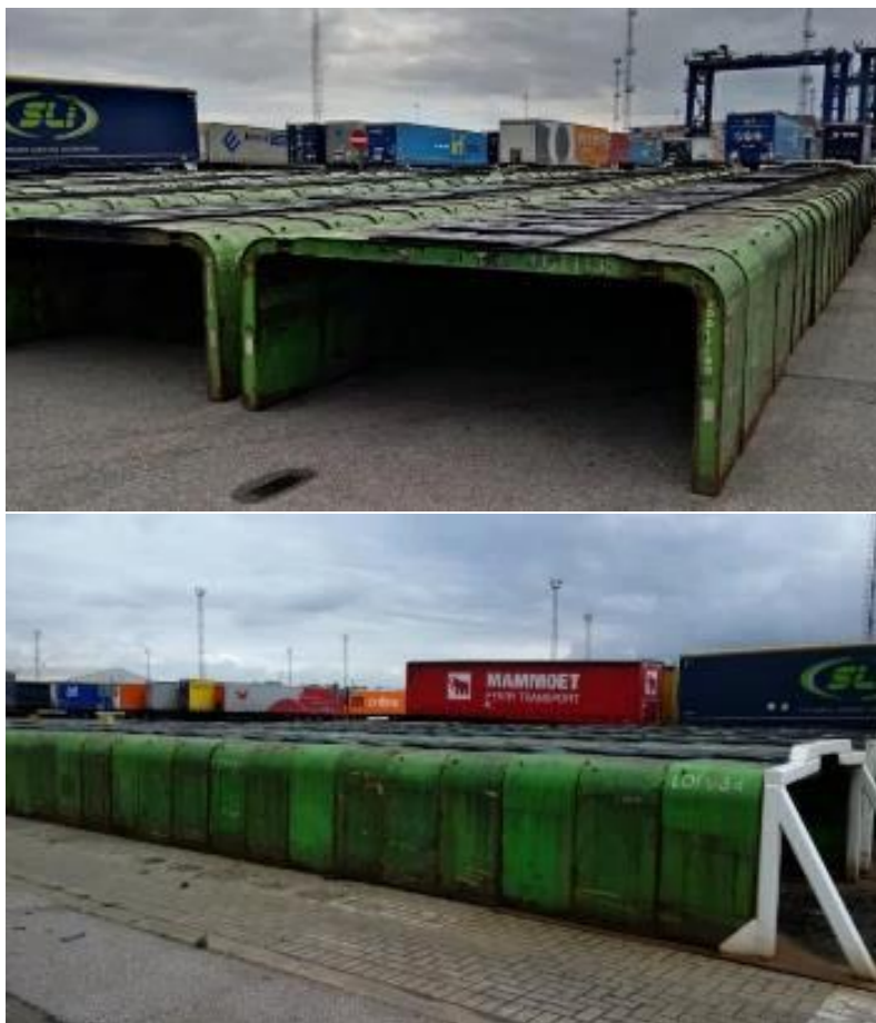
Figure 5. The pictures above show a purpose-built SAT storage area
